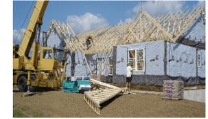
Day 1: Basement & Garage concrete poured. Basement walls, Floor System, Exterior walls, and interior walls all framed. Trusses set. Windows & Doors installed. House wrap applied.
