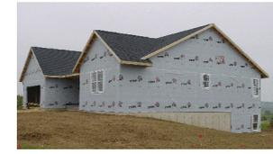
Day 7: All framing complete. Roof shingled. House wrap completed. Front porch poured. All electrical, Plumbing, & Heating rough-ins complete. Ready for inspection!
